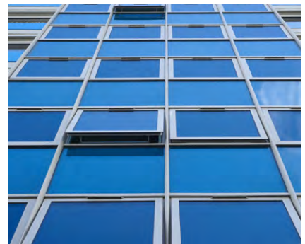
Aluminium clad curtain walling
