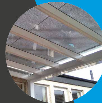
Screener Veranda Upgrade
